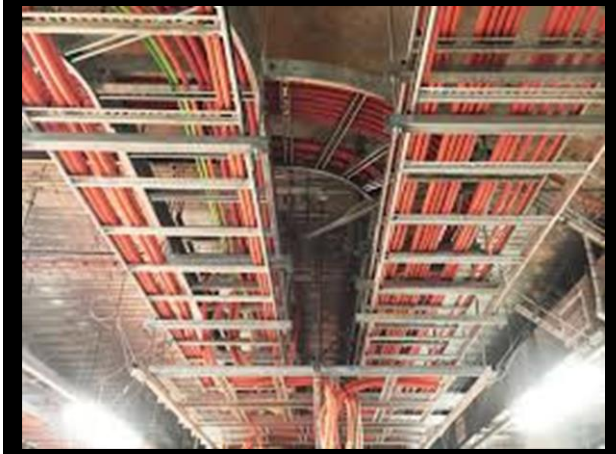
Basement Cable Tray & Submain Installation
